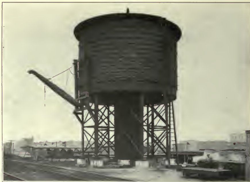
FIG. 658. FACILITIES TO BE ABANDONED. Water tank of the Chicago & North Western Railway at 16th and S. Wood streets. This tank has a capacity of approximately 77,000 gallons, is in excellent condition, and is typical of many such structures within the proposed limits of electrification. In the event of electrification, it would be rendered worthless to the railroad in its present location.
